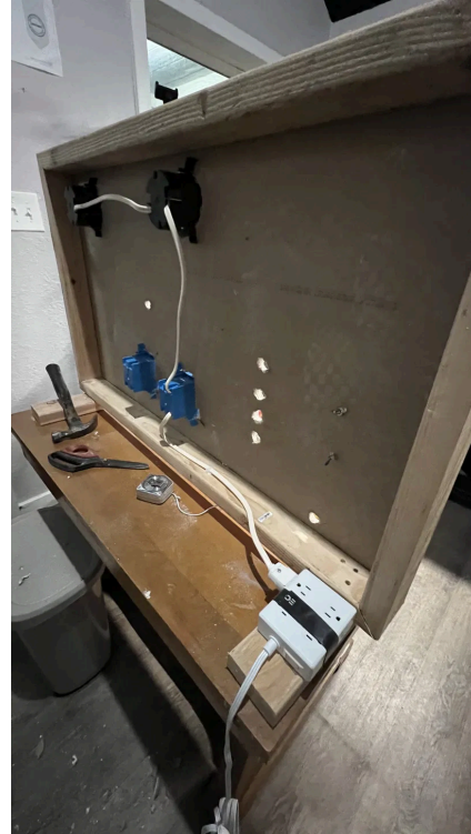
Rear reference — old-work boxes, cable paths, and back-side access before final wiring.
